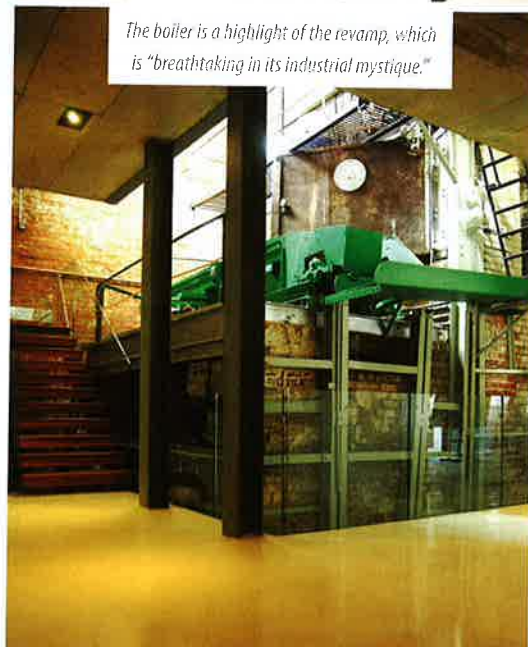
The foyer with its prominent glass floor.
