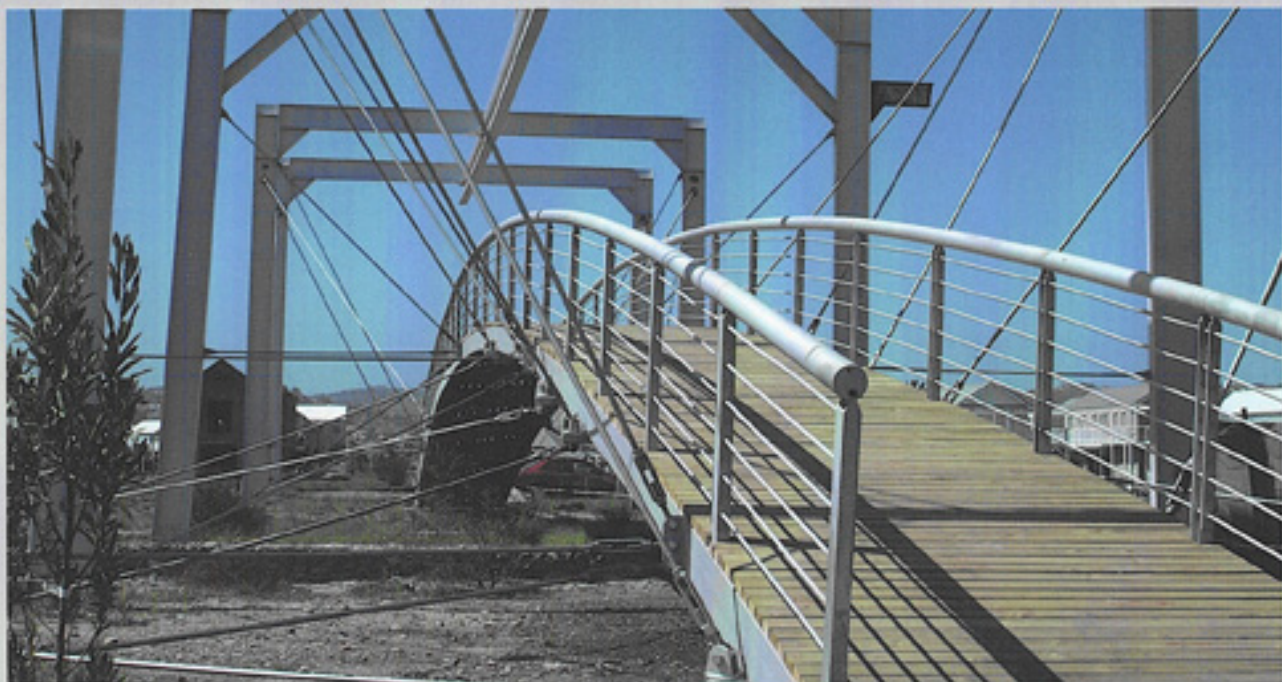
The Monorail Bridge was designed to let small boats on the channel through.
