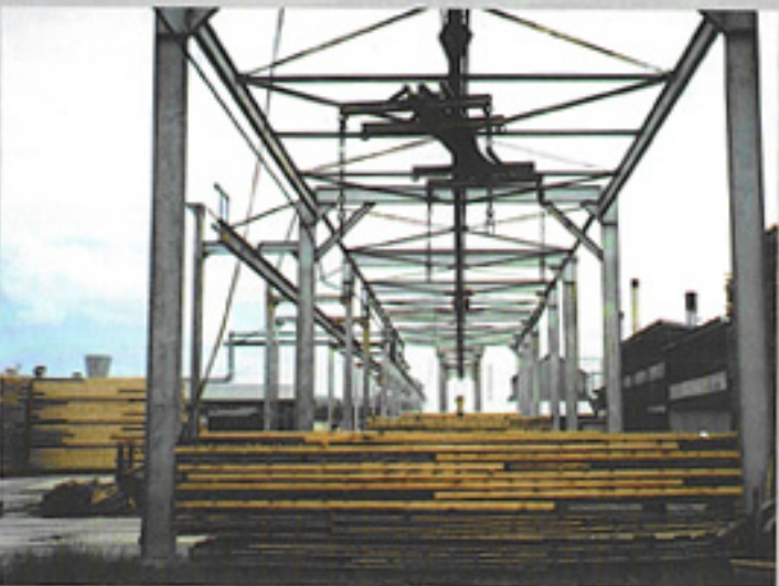
The gantry when it was still in use.
