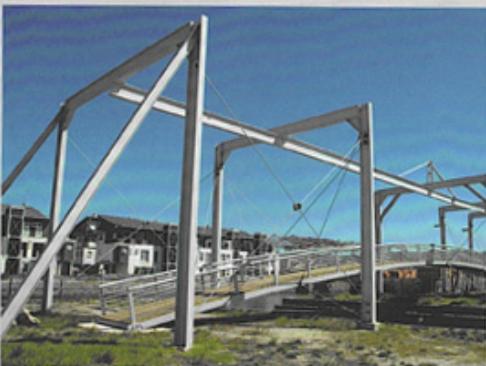
The new bridge hanging from the existing portal frame.
